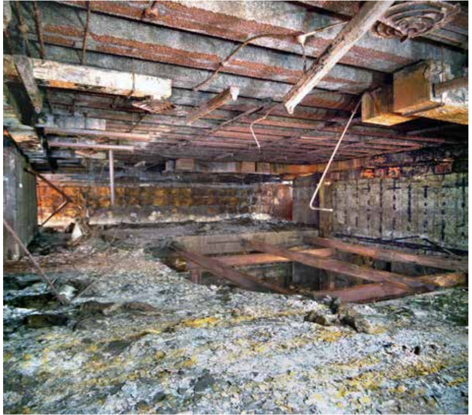
The top floor of the R4 operations room in 2001 showing the damage caused by the fire. Before the fire the well has been floored over with timber. Photo Nick Catford
